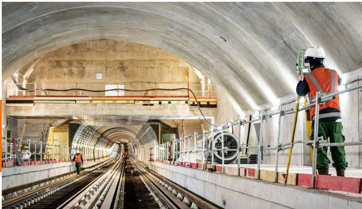
Metro line 4 extension work site.
