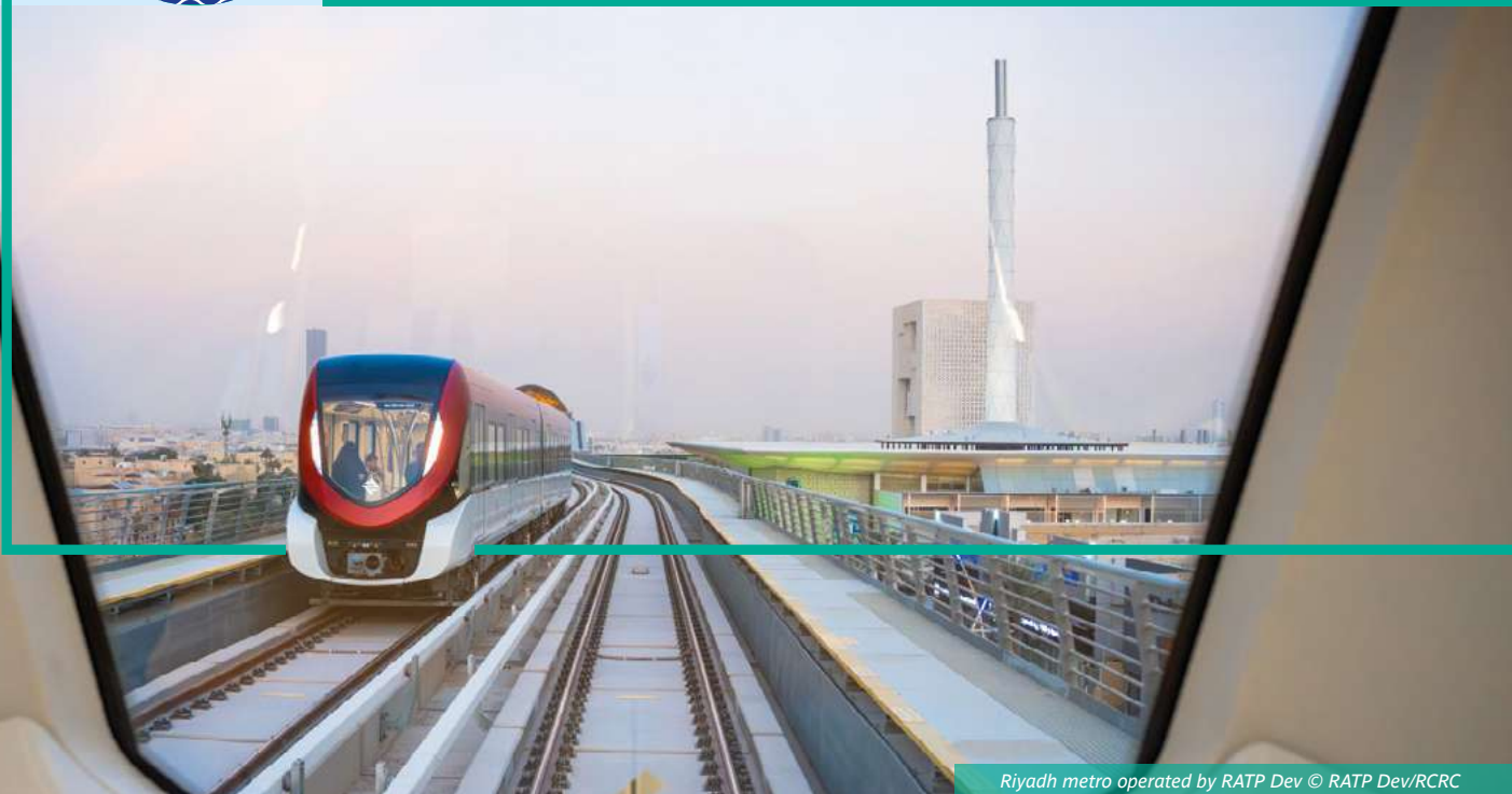
Riyadh metro operated by RATP Dev © RATP Dev/RCRC
