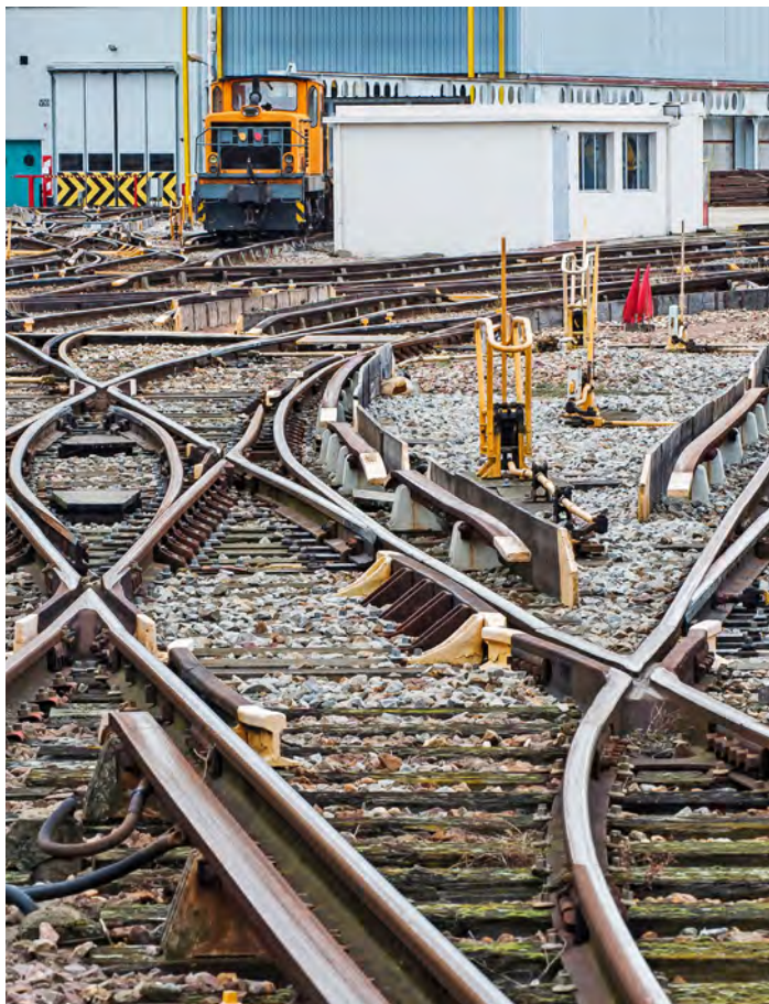
Tracks and switching systems at Villette maintenance center in Paris.
