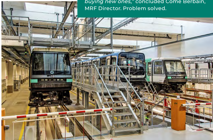
Three generations of rolling stock at the metro line 14 maintenance and depot center in Saint-Ouen.
