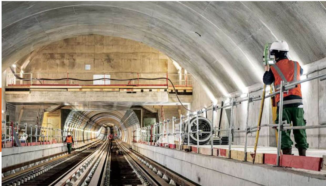
Metro line 4 extension work site.
