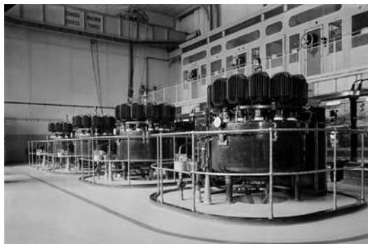
Machine room at the Auteuil substation (Paris' 16 th arrondissement), designed by architect Paul Friesé in 1912, and listed today as a historical monument.
