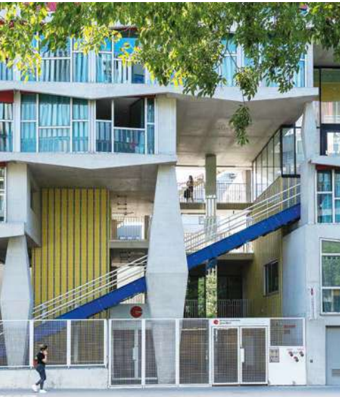
Housing units at the Ateliers Jourdan-Corentin-Issaire maintenance workshops (Paris' 14 th arrondissement).
