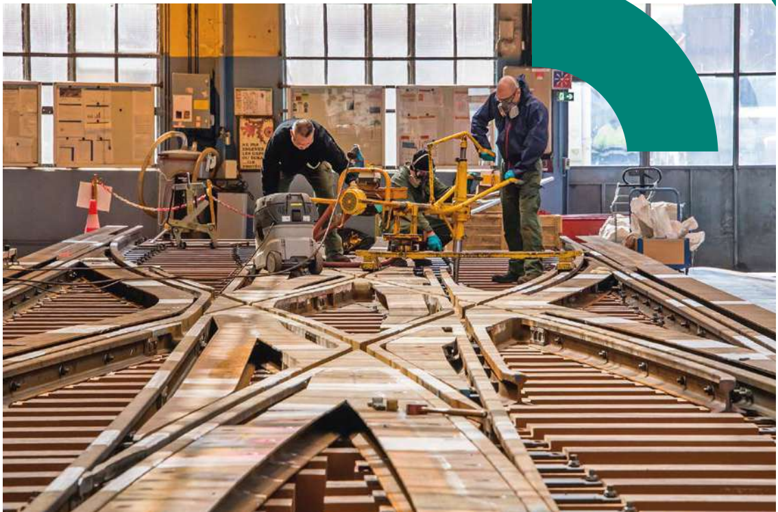
The assembly of track systems are first trialled at the Ateliers de la Villette before being laid.
