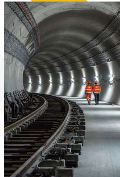
Metro line 14 extension works.
