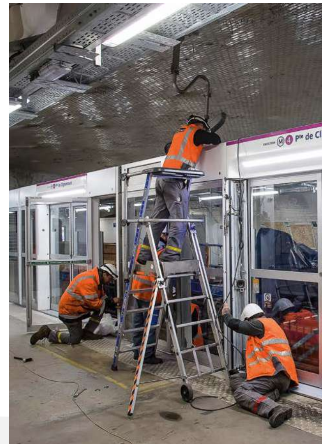
Installation of platform screen doors on metro line 4.
