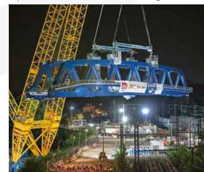
Replacement of the Chartres and Gallardon bridges.
