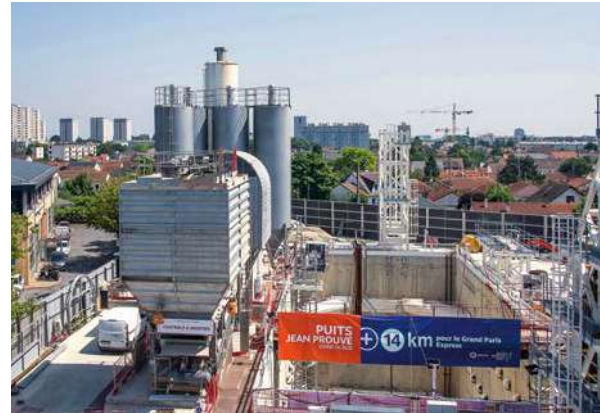
Tunnel boring machine (TBM) launching shaft in L'Hajj-les-Roses, metro line 14 southern extension work site.
