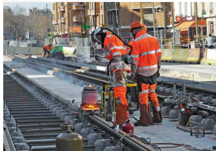
Tram line T3b extension work site.
