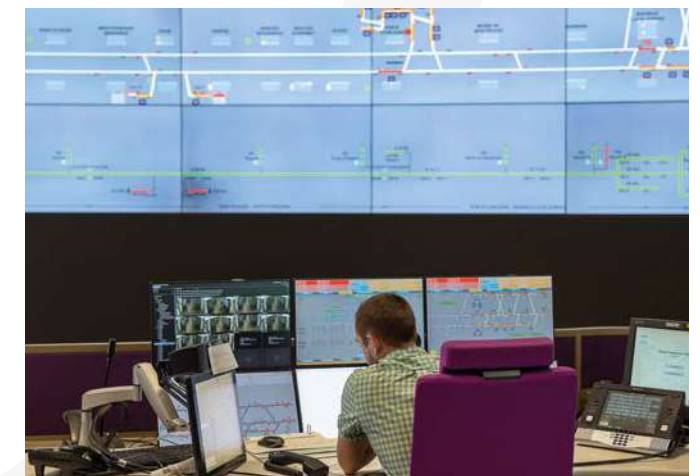
Metro line 4 central command post.
