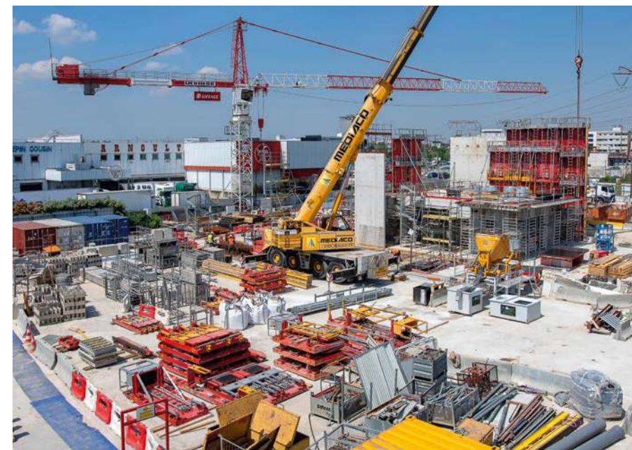
Metro line 14 southern extension work site.
